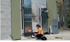
The next step is to install the mineral wool board to insulate the cell and to place the anchorings, profiles and cladding for the ventilated façade.
